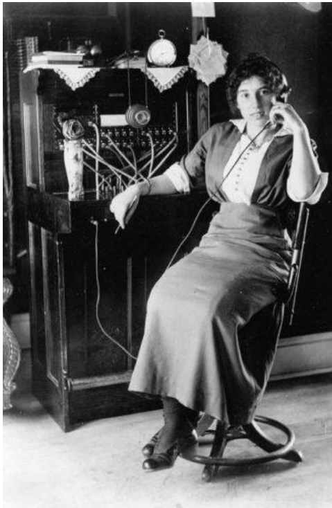
An early telephone exchange
